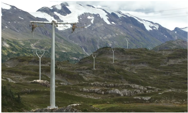
(Figure 15: The 35-mile-long, 138 kV overhead transmission line that conveys hydroelectric power to the Brucejack Mine in northern British Columbia. Source: Rokstad )
